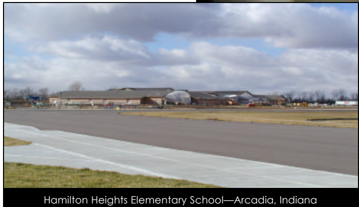
Hamilton Heights Elementary School—Arcadia, Indiana
